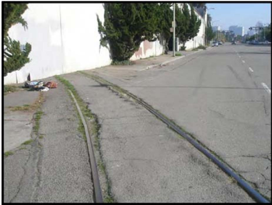
Photo IV.1: Rail lines encroaching into sidewalk corridor
