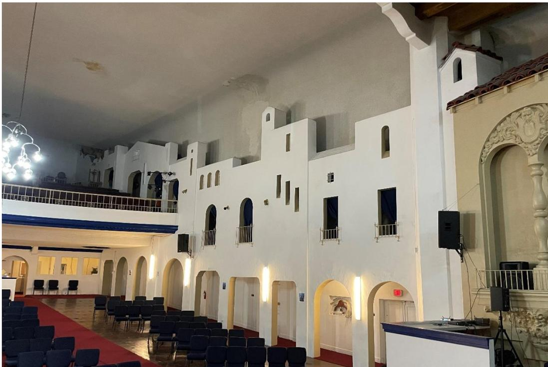
Figure 13 False façade elements at southwest wall of auditorium, balcony at left
